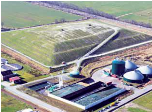
Abbildung 27: Altdeponie in Hage
